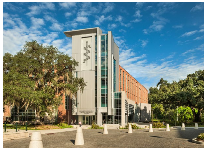
FLORIDA HARRELL MEDICAL EDUCATION BUILDING | Gainesville, FL
